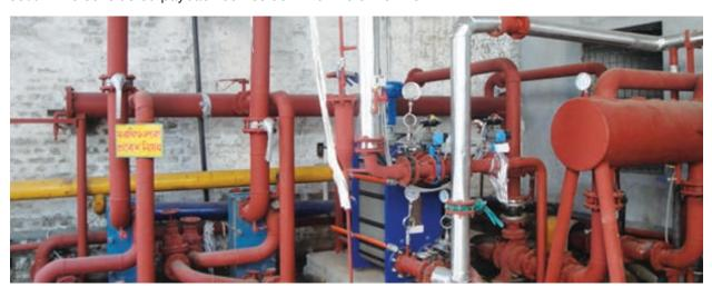
Cogeneration to recovery of heat from the Jacket Water of a Captive power Generator set for use as process heat
