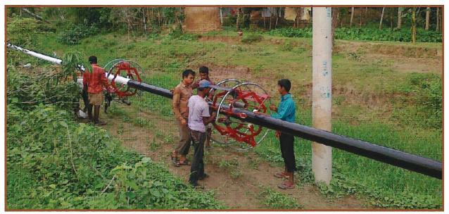
Coating and wrapping works of newly constructed 8" dia pipeline from Noyapara to Jogodispur under JGTDSL
