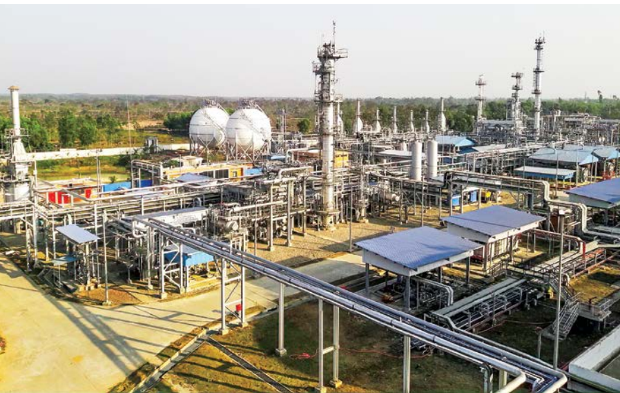
Rashidpur CRU Plant of SGFL
