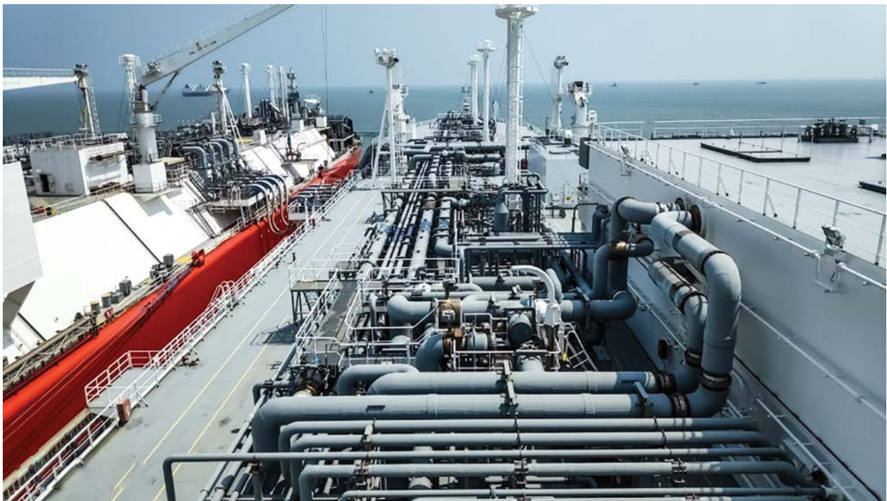
Ship to Ship (STS) LNG Transfer Operation
