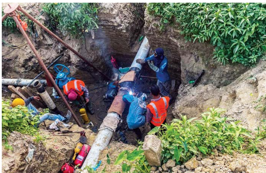
Maintenance work in Cumilla by BGDCL
